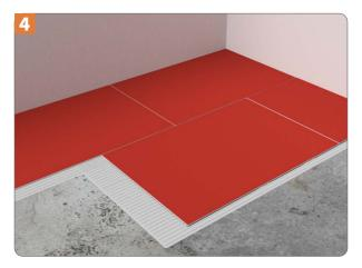
Ultralight should be laid on the freshly applied ribbed bed and thoroughly bedded in to ensure that no voids are left beneath the boards and they are solidly supported. All boards should be laid with staggered joints.
