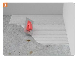
Ultralight should be installed using a flexible, cement-based adhesive. The adhesive should be trowelled out and combed through using a 6 mm x 6 mm (¼" x ¼") square notch trowel to give a ribbed bed, any slight depressions in the subfloor being filled by the mortar.
